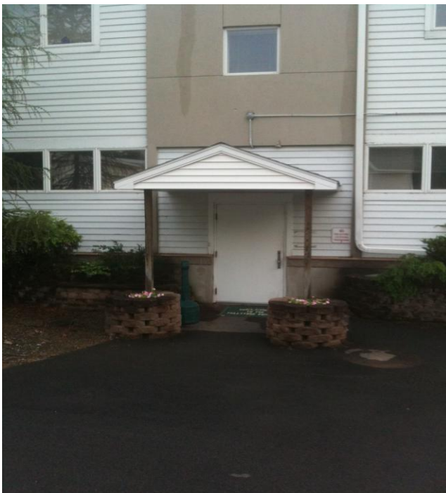
Enter the building here please, around back of bldg!
